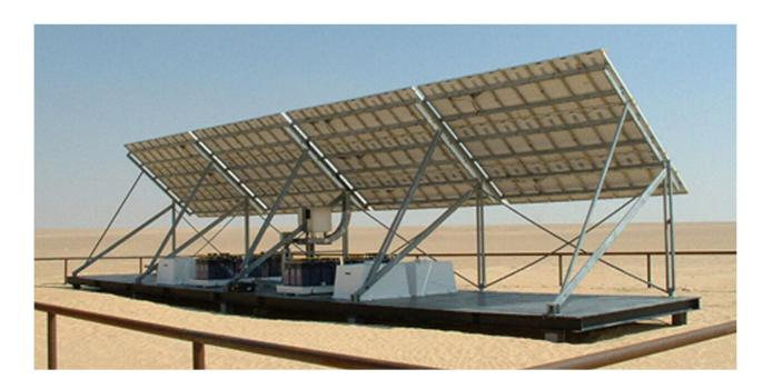
The structure provides high level mounting for the modules, with an adjustable tilt angle. Each kit is supplied with all fasteners including ground anchor bolts and a comprehensive manual. This structure has been in use for over 15 years and has provided power for many systems including telecomms, cathodic protection and remote power.
